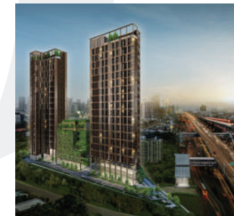
LANDMARK AT KASERT TSH STATION Bangkok
